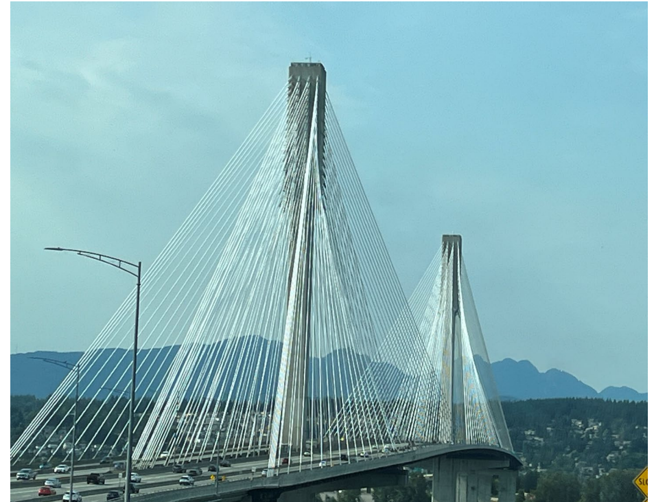
Port Mann Bridge, Vancouver, BC
